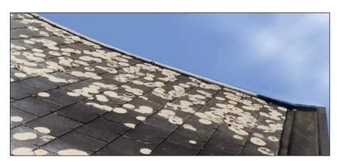
Roofs made of artificial slates, tiles, cement bound plates etc., are very much subject to air pollution, acid rain and the adhesion of algae and moss. These environmental factors affect the substrate and without any protection this substrate will continue to be subjected to these natural elements. This might eventually cause the total destruction of the roof. It can also cause the release of harmful asbestos fibres, a major danger to our health.
